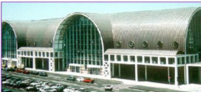
AIR TERMINAL Ostiense
